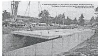
Figure No. 02 - Culvert with Hinge Joint at Top
